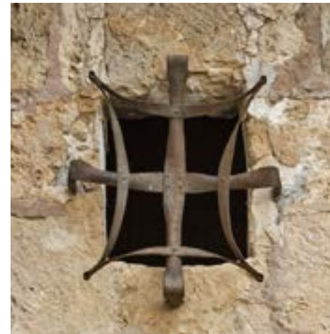
Window with a cross-shaped wrought-iron grille designed by Antoni Gaudí.
