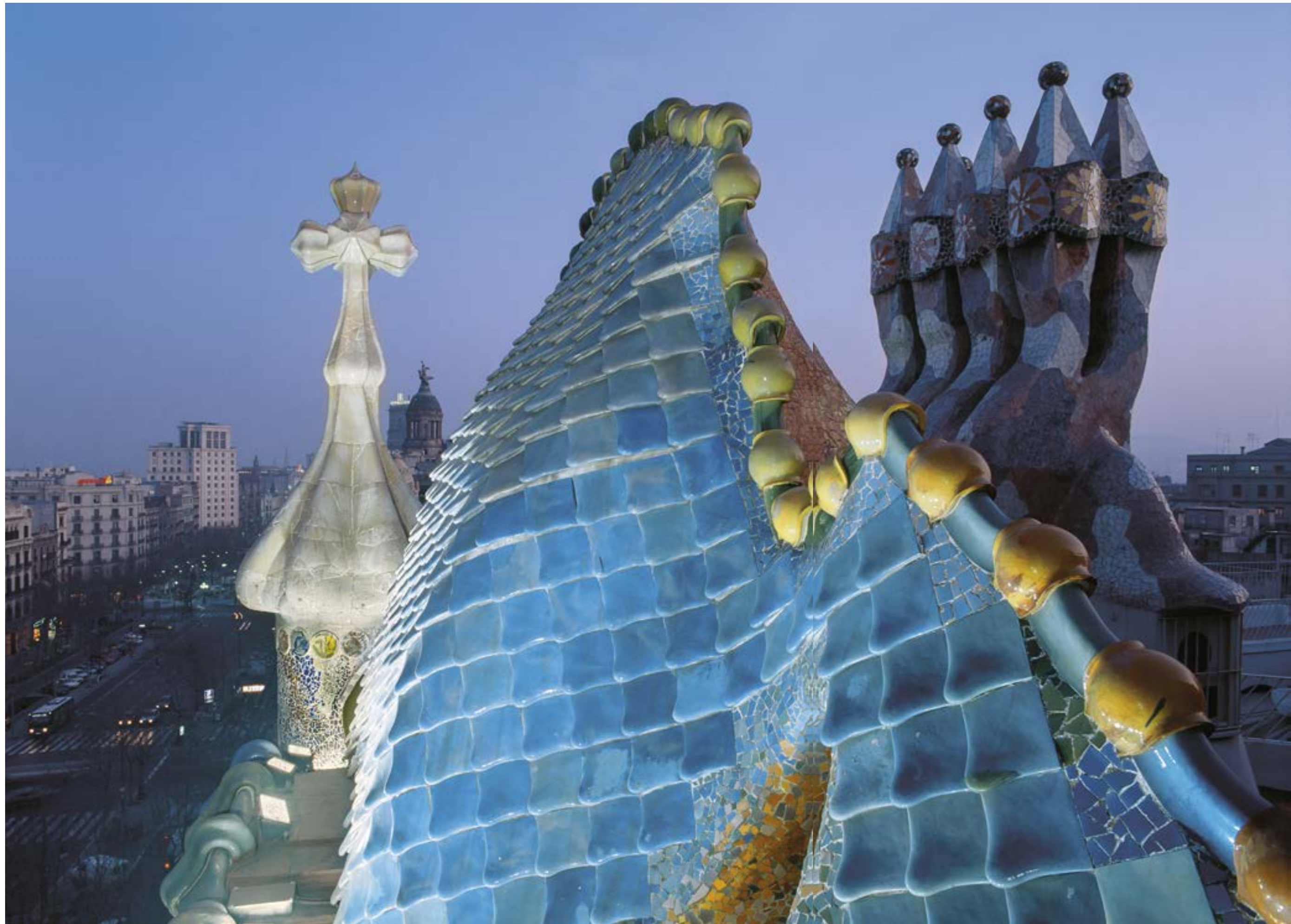
Rooftop of the main façade clad in ceramic pieces in the shape of scales. The ridge is made more eye-catching with semi-spherical pieces placed over cylindrical ones.
